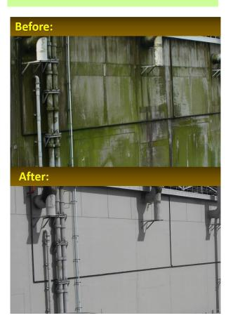
A Nano Technology coating system that incorporates nano TiO2 (titanium dioxide) and other proprietary nano particles for maximum anti algae effect.
